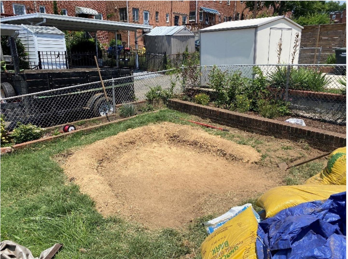
If compacted clay soils are not strong enough to keep the berm solid, stable, and level, you may add rocks or bricks around the berm to help strengthen it (see picture above in Berm section). You should not plant your berm or allow plants to grow on it.
