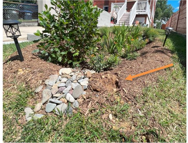
The berm of this rain garden is not compacted enough and overflowing water is eroding the berm.
